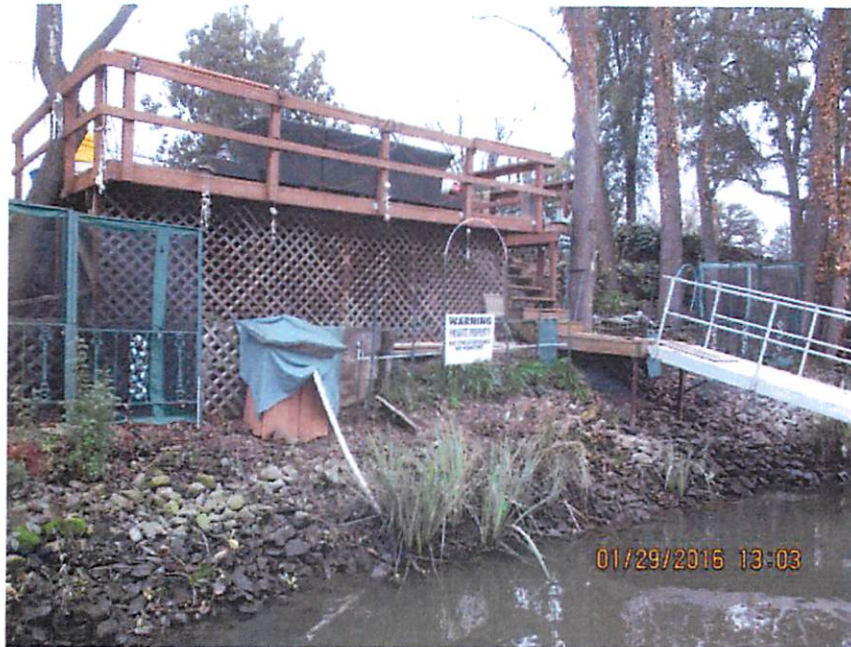
The waterside view of the levee. Conversations with Mr. Schantin revealed that the tides get as far up the bank as the small pump station shown in the middle of the photo.
