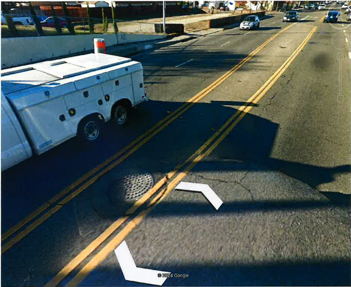
Manhole 4 is the southernmost of two manholes north of the Pershing Ave. Bridge and is currently not being utilized on this project. This is likely where the submarine portion of the sewer line exits Smith Canal and returns to the subterranean alignment.
