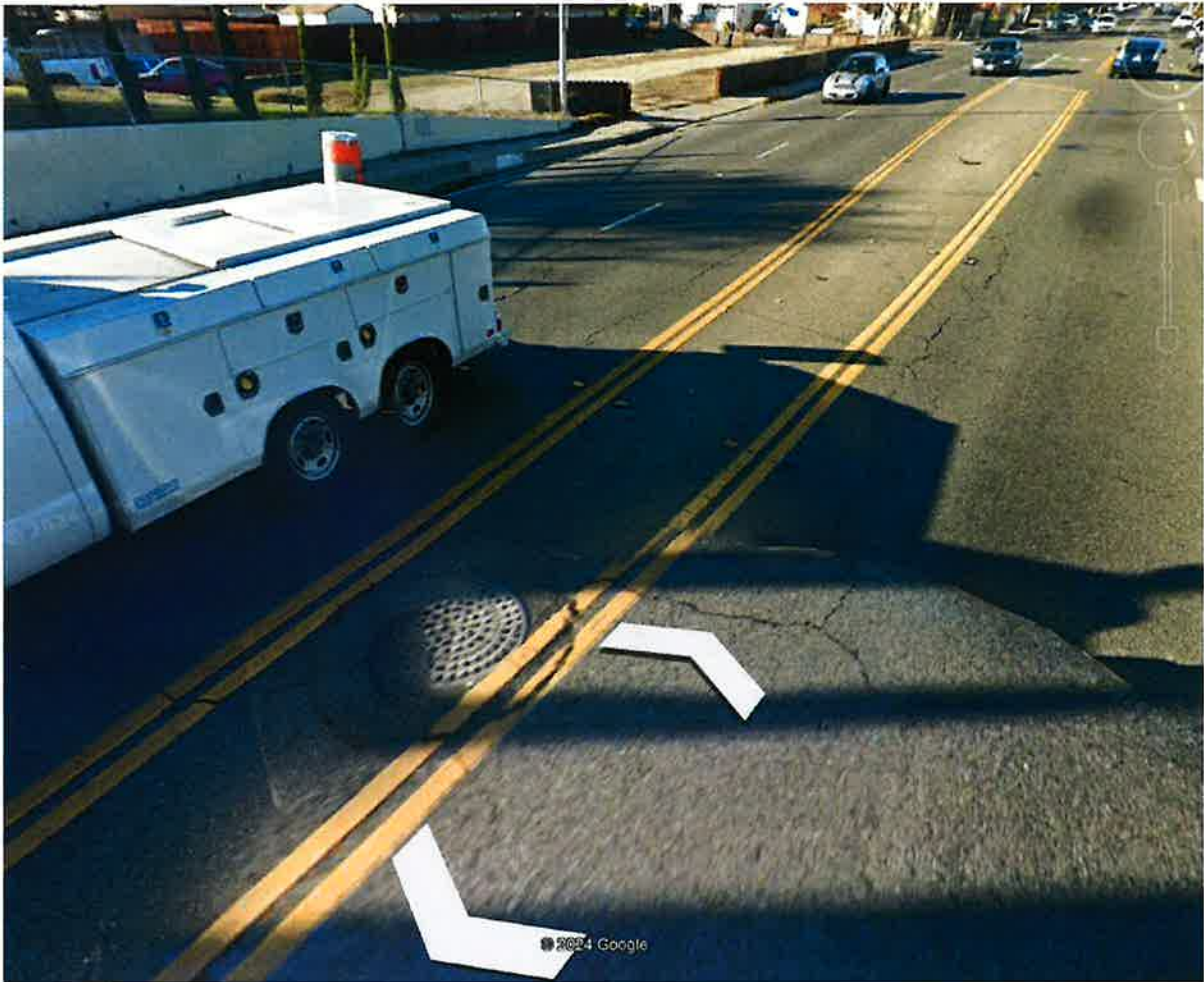
Manhole 4 is the southernmost of two manholes north of the Pershing Ave. Bridge and is currently not being utilized on this project. This is likely where the submarine portion of the sewer line exits Smith Canal and returns to the subterranean alignment.
